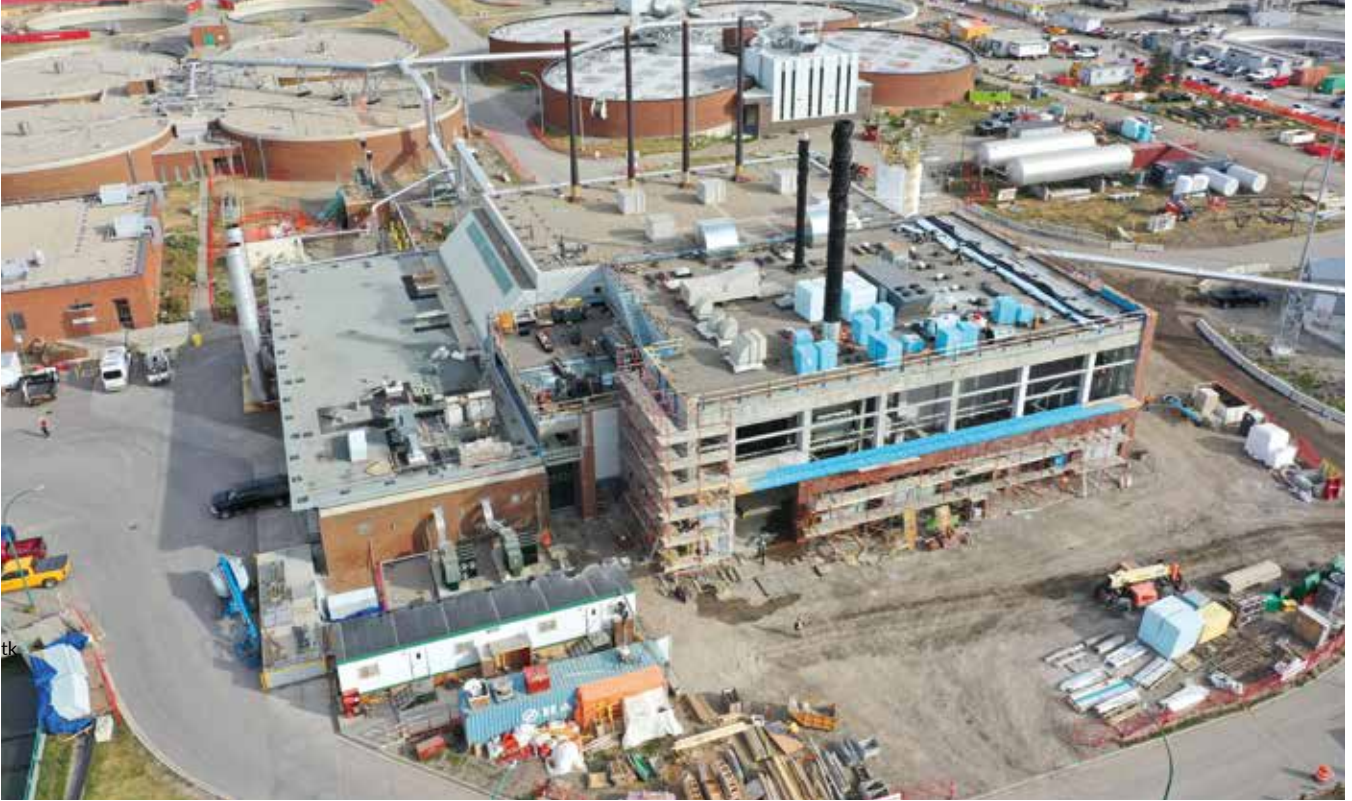
Bonnybrook Wastewater Treatment Plant
