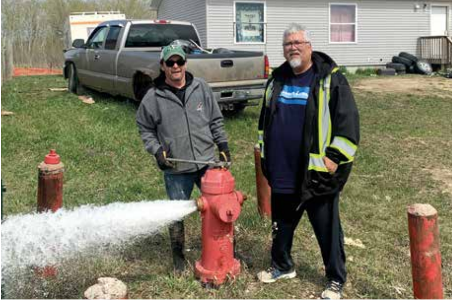
Deon Hassler and operator, Dale Desnomie (left), flush water mains and check hydrants on Peepeeekisis First Nations.
