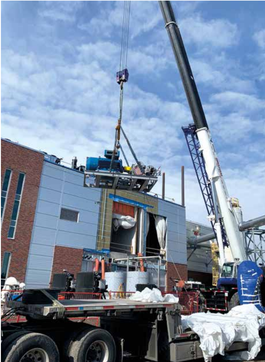
The steam turbine generator will be used to create additional plant or will feed the future thermal hydrolysis process facility.
