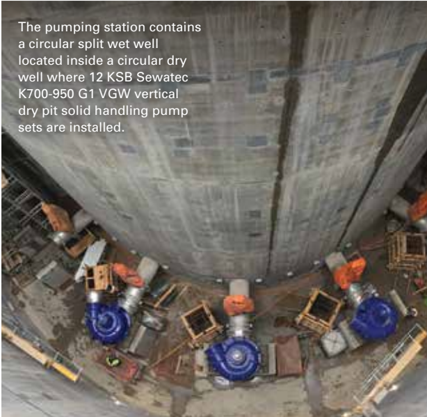
The first of the pumps being installed and anchored to their mountings.
