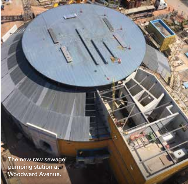
The pumping station contains a circular split wet well located inside a circular dry well where 12 KSB Sewatec K700-950 G1 VGW vertical dry pit solid handling pump sets are installed.
