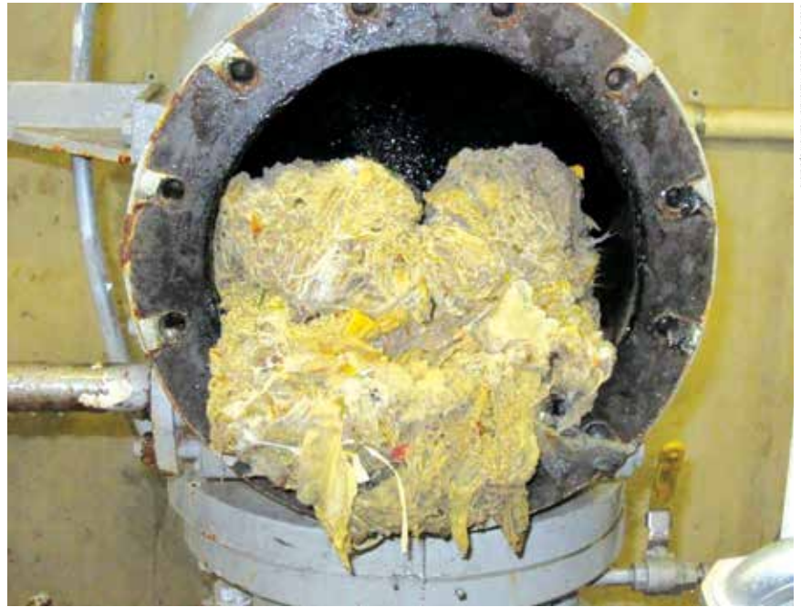
Credit: City of London Wastewater Treatment Operations
