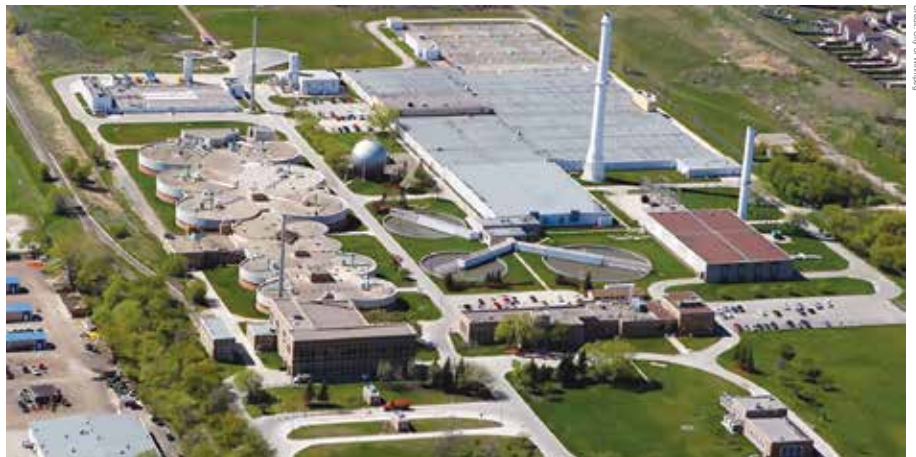
Credit: City of Winnipeg
