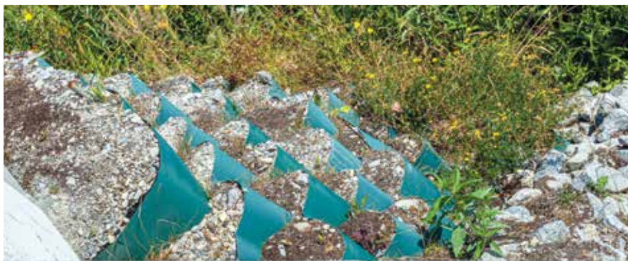
The Region of Peel is mitigating the potential impacts of polluted runoff from an infrastructure project with a living wall.
