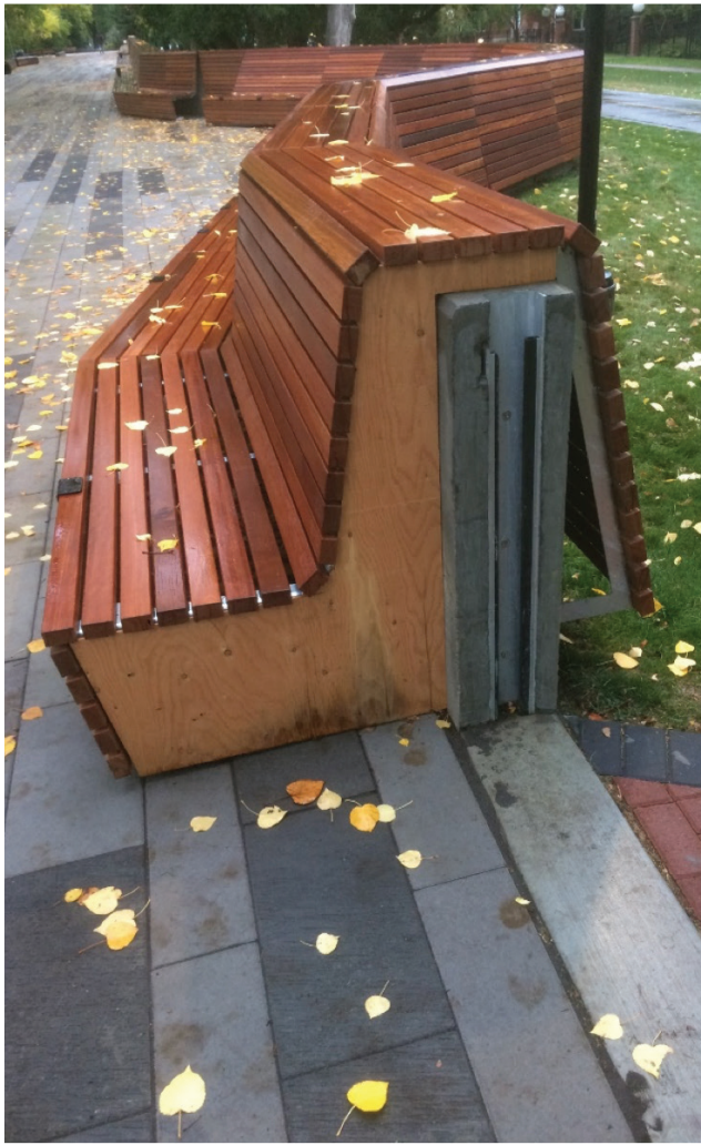
Figure 1 - Concrete section of West Eau Claire Flood Barrier showing aluminum guides where stop-logs are placed during a flood emergency
