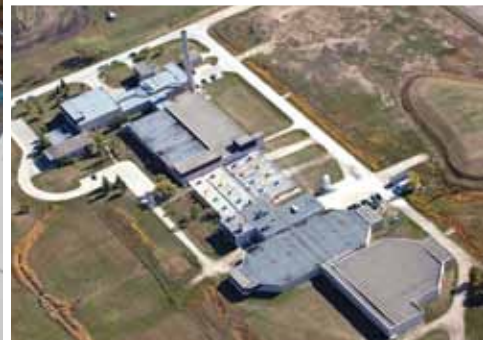
The secondary clarifiers that are being constructed and the second one
