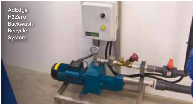
AdEdge's arsenic and iron removal system.
