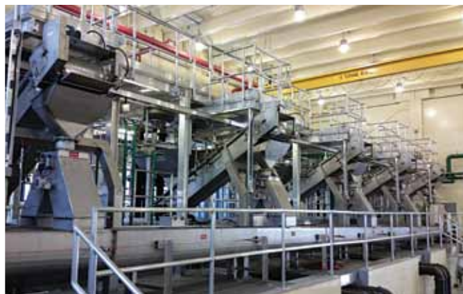
The HeadCell grit removal system from Hydro International is based on the principles of advanced grit management.
