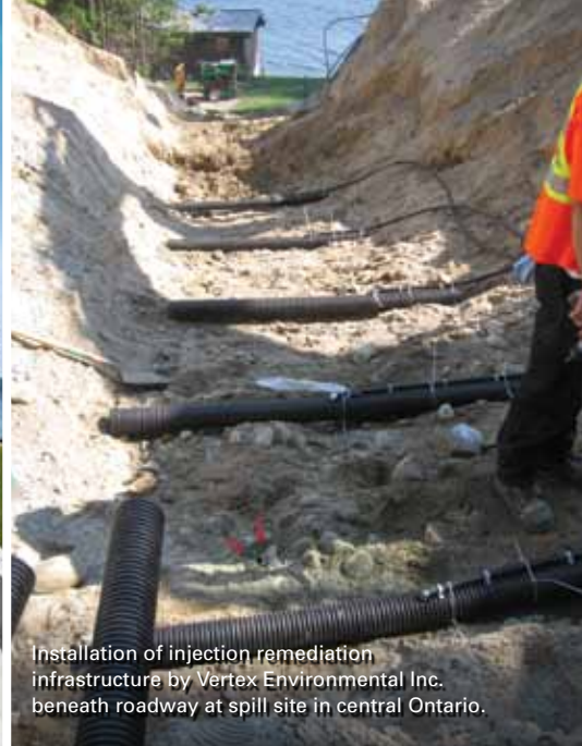
Remediation crews installing injection infrastructure adjacent to Lake Ontario in Toronto's Portlands district.
