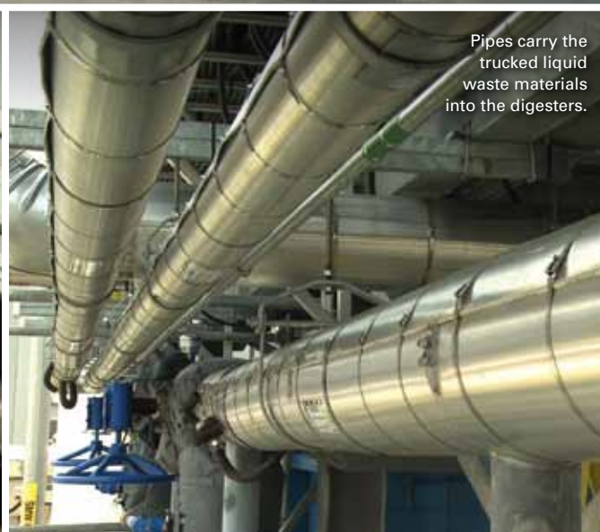
Energy-rich materials such as fats, oils, and greases from restaurants and food-processing plants are fed into a co-digester to increase energy production. This generates revenues through tipping fees and prevents these materials from clogging the sewer pipes.
