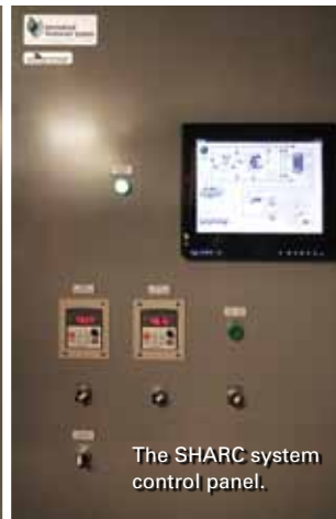
The system has direct digital controls with a touch-screen interface, data logging, and remote monitoring capability.
