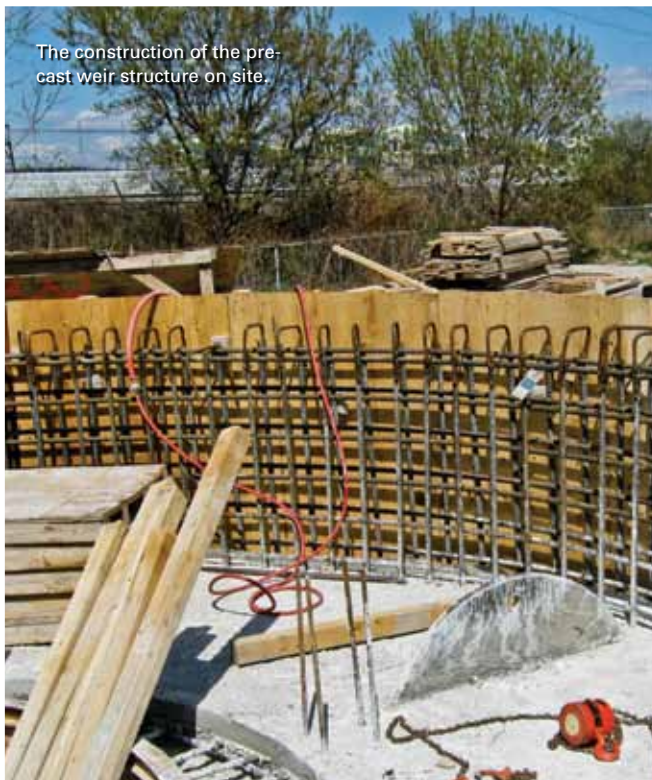
The main storage shaft prior to the pre-cast weir tower assembly.
