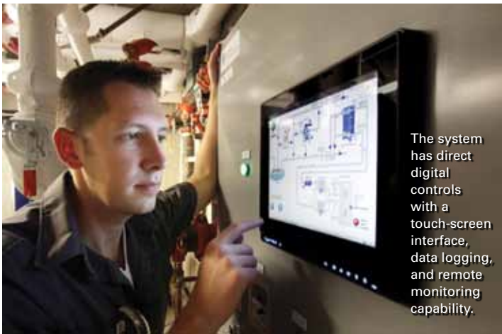
International Wastewater Systems' SHARC sewage heat recovery system is fully sealed, odour free, and maintained by factory-trained personnel.
