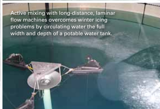
Ice buildup in potable water storage tanks can cause structural damage and water leaks, leading to extensive maintenance and expense.
