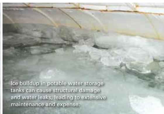
Active mixing with long-distance, laminar flow machines overcomes winter icing problems by circulating water the full width and depth of a potable water tank.
